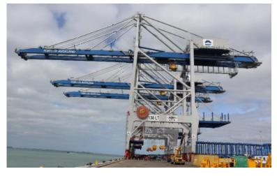
**Hatch Platforms** have now been installed on all container cranes – these allow the ship's hatch covers to be stored above the ground, freeing up space around the cranes for container handling.
